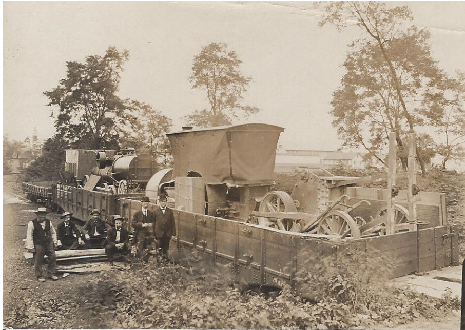
The heavy equipment for the Dehaven Road reconstruction was brought to town by railroad. The cars are on a side track below Rutters (now Sensenig Feed Mill). In the background on the left is the steeple to St. Stephen Reformed Church, and visible on the right side is Kinzer's Lumber Yard (now Musselman's) and the Silk Mill.
