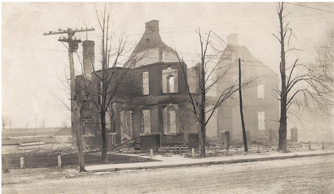
View from the intersection of Main Street and Kinzer Avenue showing the remains of the home shortly after the fire was extinguished (burned out). The smoke still lingers and there are still walls in danger of falling.
