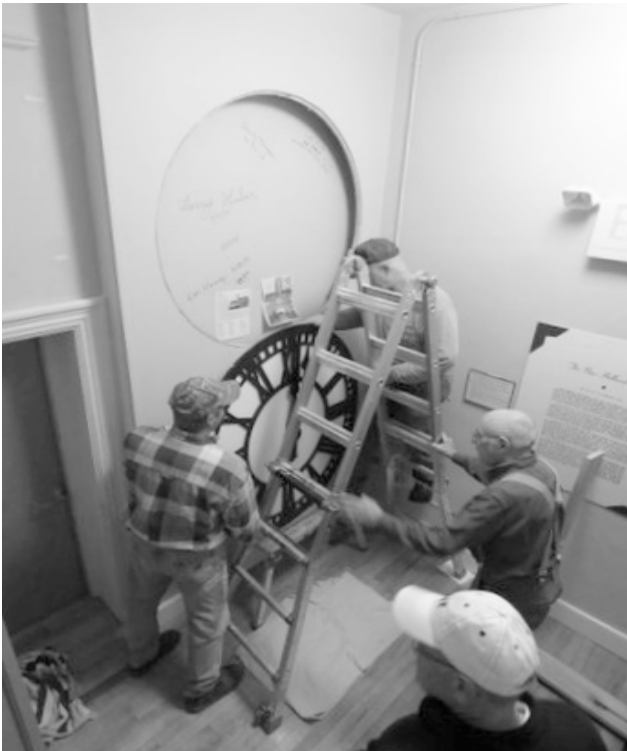
Clock being prepared to be lifted into place
